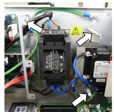
(8) Mount the five screws on the side of the chassis.
